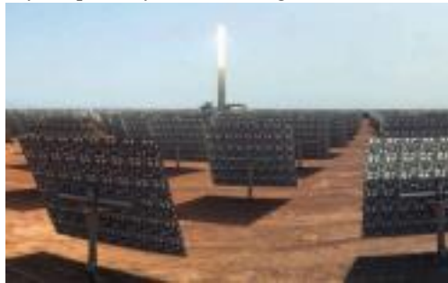
Figure 3. Heliostats installed at Noor III in Morocco; Source: Roadmap to Advance Heliostat Technologies for Concentrating Solar-Thermal Power, link to reference ?
